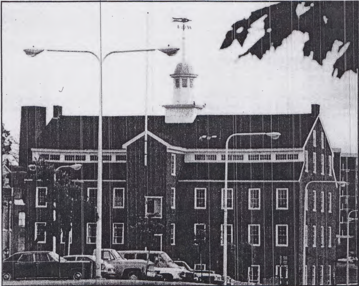
The Belknap Mill in the early 1970's with exterior renovations complete.
