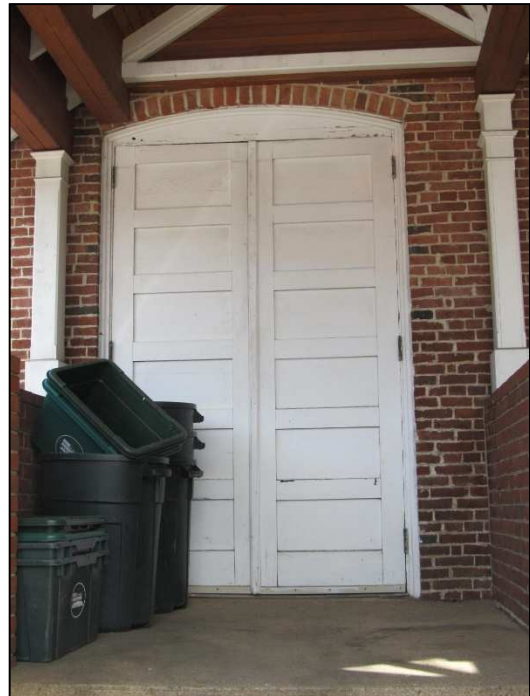
Figure 6: Southwest door to Belknap Mill.
