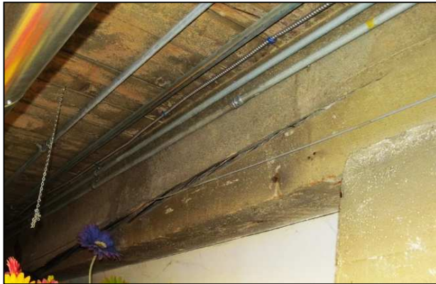
Figure 12: Example of checking in beam
