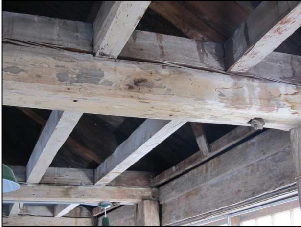
Figure 22: Checked beam, 4th floor
