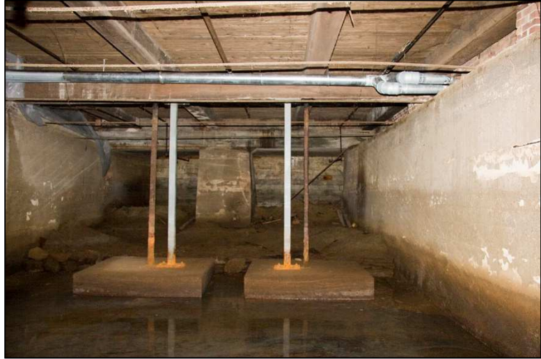
Figure 11: Sluiceway beneath east portion of Belknap Mill
