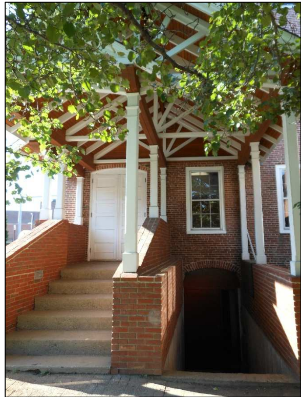
Figure 8: Portico at southwest corner of Belknap Mill
