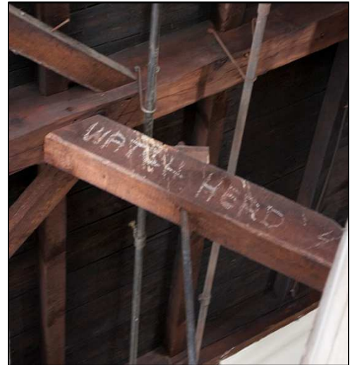
Figure 15: Graffiti on attic strut.
