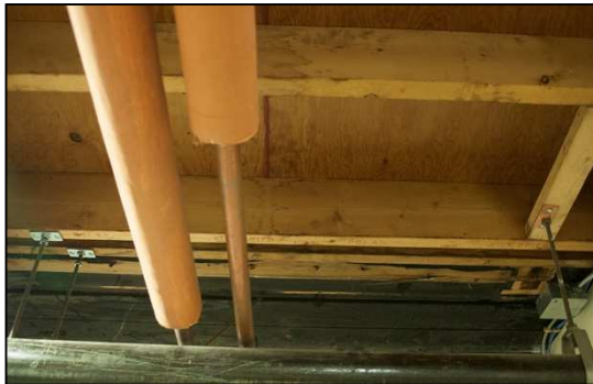
Figure 18: Modern flooring at southwest corner of Belknap Mill
