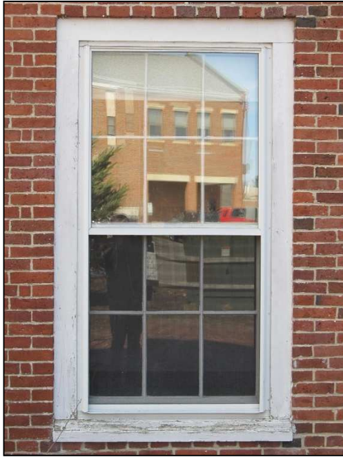
Figure 4: Typical 6/6 wood window.
