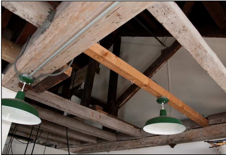
Figure 14: King post truss, attic.
