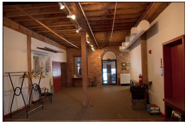
Figure 9: Lobby, facing south
