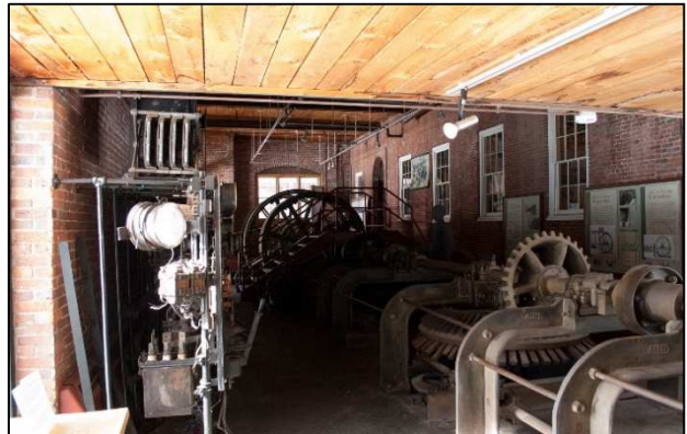
Figure 23: Facing west in Power House, present day.
