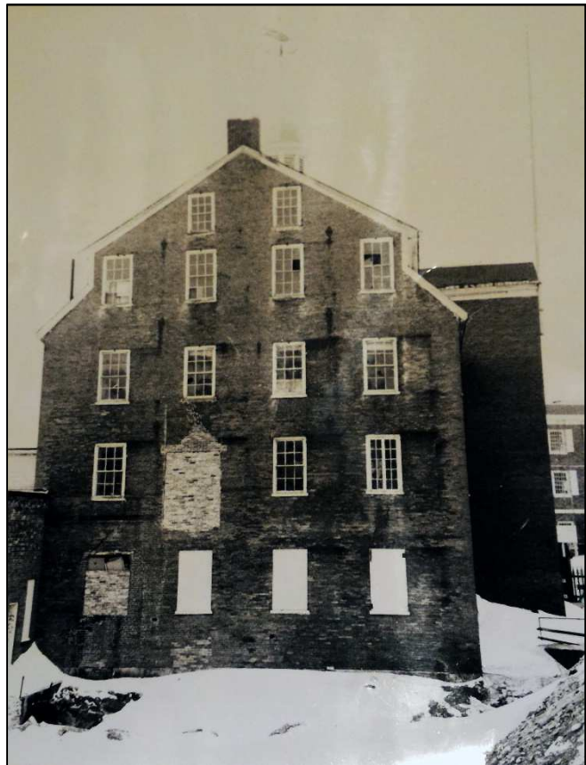
Figure 14: East elevation of the Belknap Mill from site of Esty Mill ca. 1971. (From the Collection of the Belknap Mill Society)
