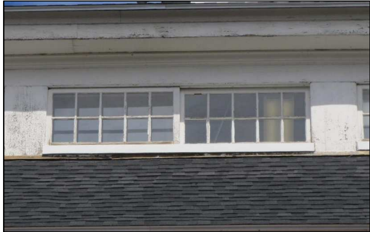
Figure 5: Typical clerestory window.
